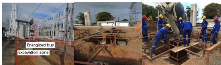
4c) construction of oil basins; 4d) fire wall construction; 4e) grounding (exothermic welding)
