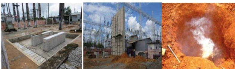
4c) construction of oil basins; 4d) fire wall construction; 4e) grounding (exothermic welding)
