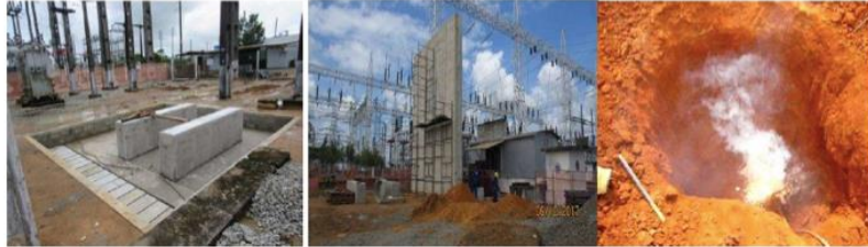
Figure 4 The construction activities
